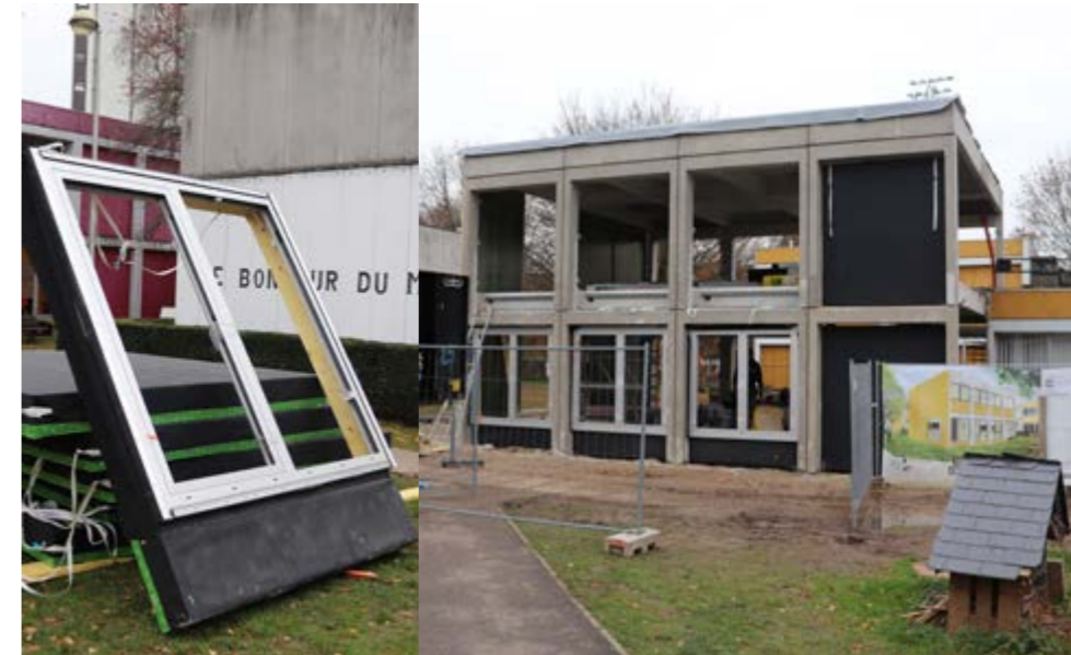
Figure 105: Eléments de façade non porteurs (Source: Architectural Engineering, VUB)
